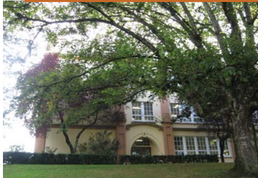
1. East wing from 10th Avenue
