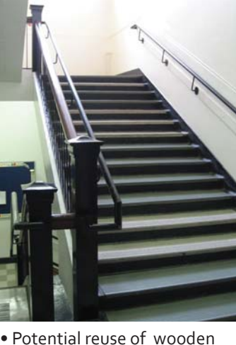
• Potential reuse of wooden handrails, steel banisters and newel posts
