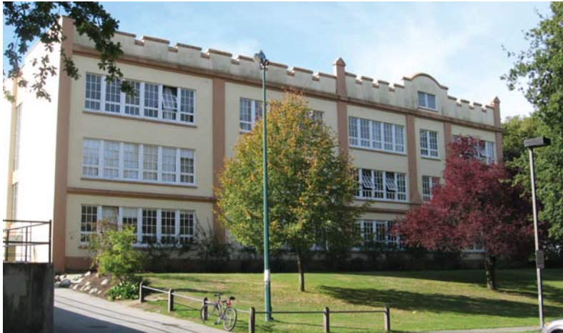
• Retain three-storey east, north and west facades of the 1927 building (repair and repaint to original colour scheme)
