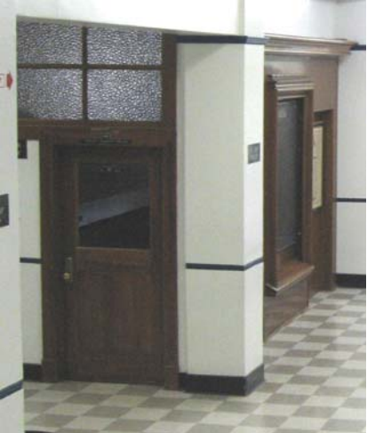
• Potential reuse of interior doors and wood surrounds
