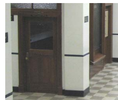
• Solid wood-paneled doors with wood surrounds and single-pane transoms
