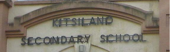
• Retain sign over main entrance
