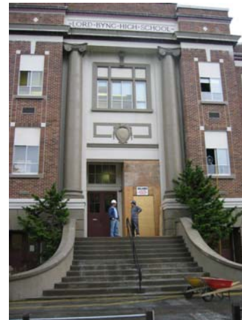
Minimize Disruptions during Construction
